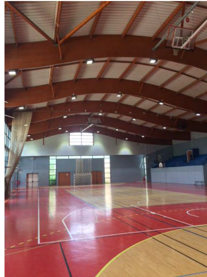
Installed Luminaire: ECO-FLB200-U-T5M
